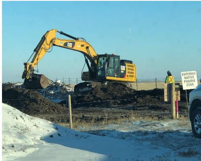
STRIPPING TOP SOIL FROM ACCESS ROAD.
