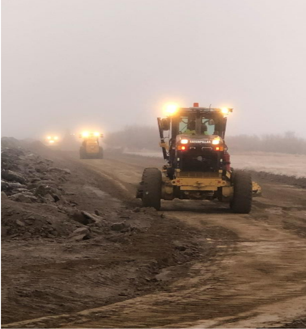
LEVELLING ACCESS ROAD WITH GRADER.
